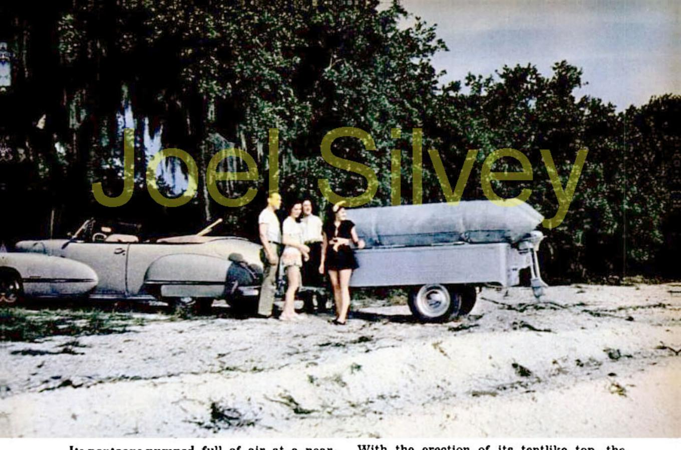
Its pontoons pumped full of air at a nearby gas station, the amphibious trailer begins to take shape. Next, the top will be opened out like a double door over the rubber-lined, canvas air bags, increasing the width of the usable space to about 12 feet.
